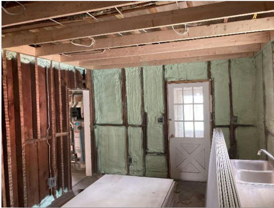
Above: Before (left) and after (right) kitchen. Strategically used spray foam to fill gaps in exterior wall insulation and to seal off the main floor from the attic and crawl space.
